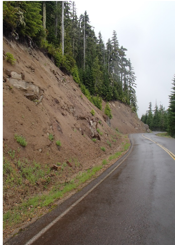
Figure 20. Rock cut where differential erosion is the dominant cause of failure. Forest Service Road 25, Milepost 30.
