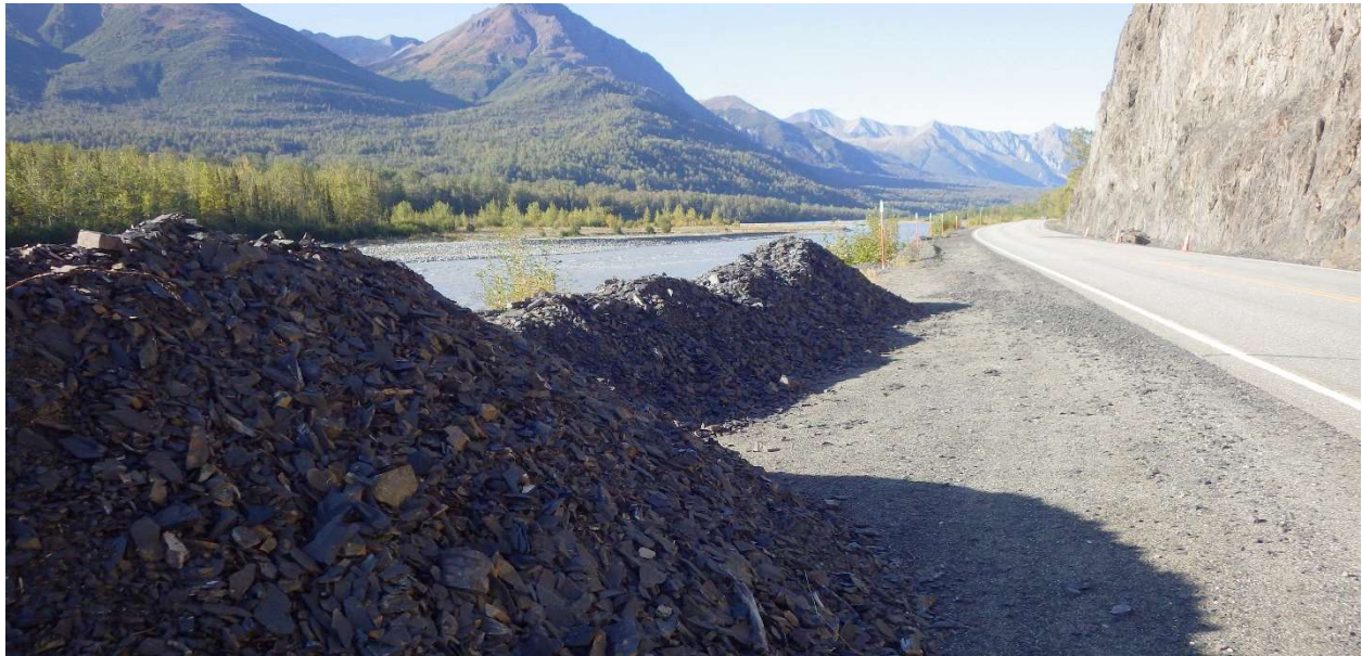
Figure 17. Constant rockfalls occur at this rock slope on the Glenn Highway in Alaska. Maintenance personnel stockpile the daily debris in this pullout for regular removal. This rock cut received a category score of 81.
